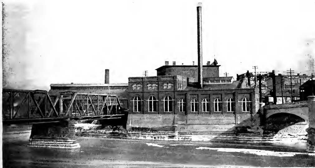
FIG. 1.—GENERAL VIEW OF POWER PLANT AT ZANESVILLE, OHIO.
